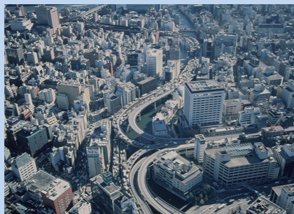
Junction constructed above a river (Edobashi Junction)
