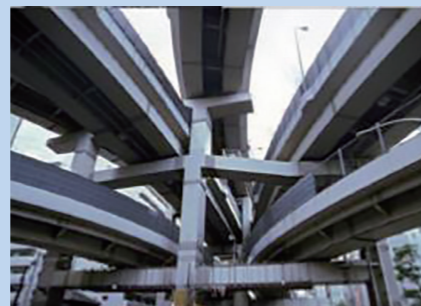
Multilayered structure (Hakozaki Junction)
