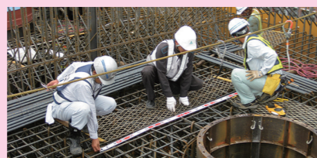
Check of rebar arrangement
