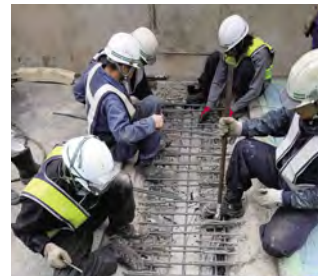
Work to eliminate expansion joints
