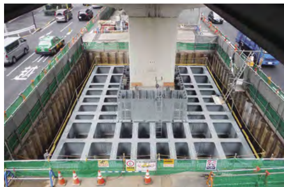
Hybrid structural footing embedded with steel grid
