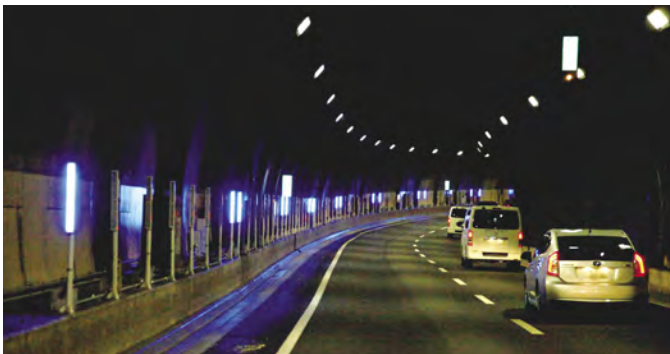
“Escort” Lights Near the Central Circular Route (Inner Route) Nakano-chojabashi
