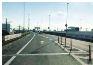
Measures to prevent driving the wrong way when merging with the main traffic flow Misato JCT
