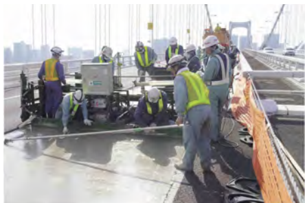
Work on preventing fatigue damage to steel floor plates being implemented
