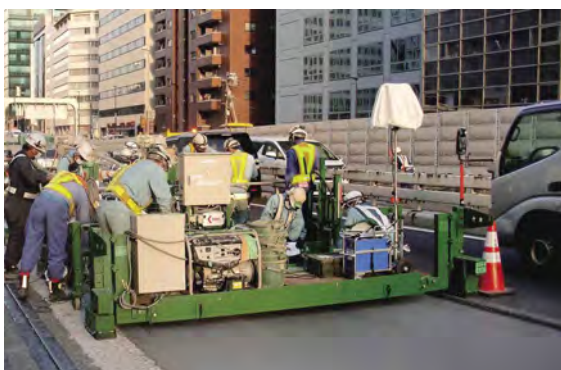
PCM paving work (Route No. 3 Shibuya Line)
