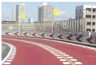
Caution-evoking painted pavement near Kiba on Route 9 Fukagawa Line
