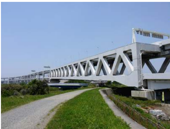
Okuma river truss bridge
