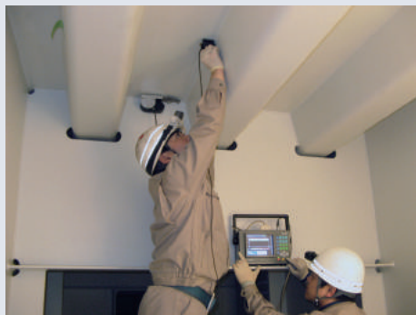
Steel plate floor Automatic Ultrasonic Testing equipment (SAUT).
