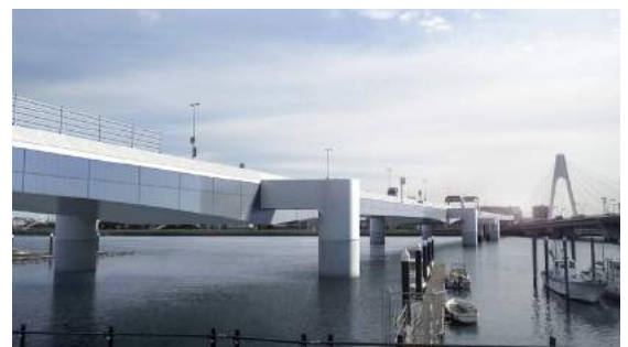
Image of the renovated Daishi bridge
