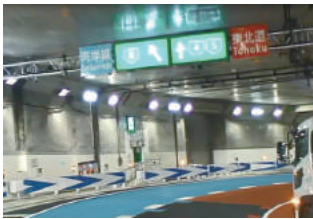
Signs and road surfaces color-coded by direction of travel at Ohashi Junction
