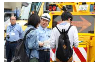
Capital express inspection / repair demonstration 2017
