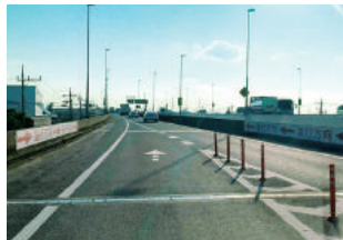
Measures to prevent driving the wrong way when merging with the main traffic flow at Misato Junction
