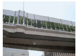
Greenery on a Nishi-Shinjuku Junction girder
