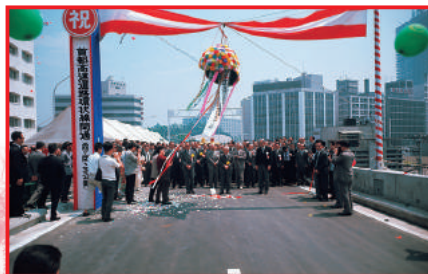
Opening ceremony for the Shiba-Koen to the Kasumigaseki section of the Inner Circular Route, 1967
