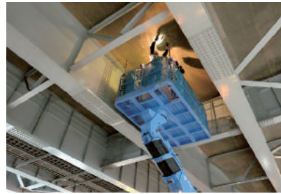
Inspection with a cherry picker
