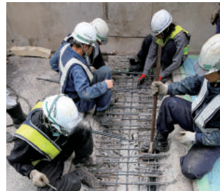
Work to eliminate expansion joints
