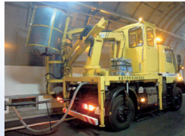
Tunnel wall cleaning
