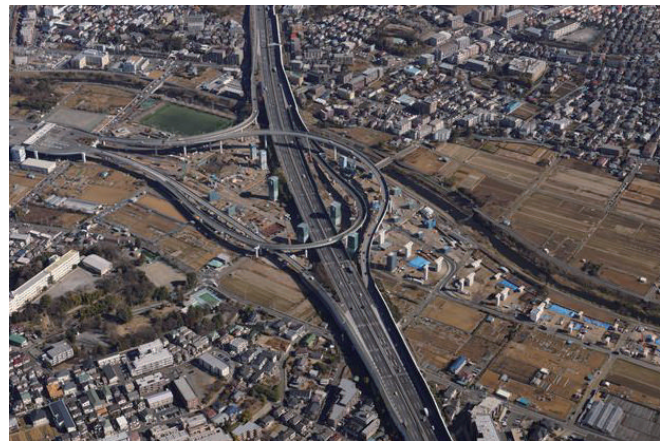
Yokohama Aoba IC / JCT (tentative) construction site
