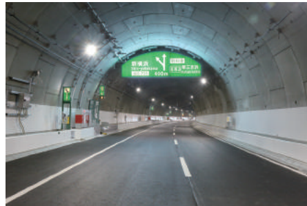
Yokohama North Tunnel
