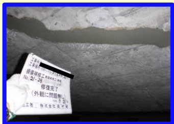
ひび割れ補修
