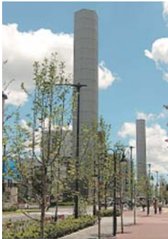
Yamate Tunnel ventilating tower.
