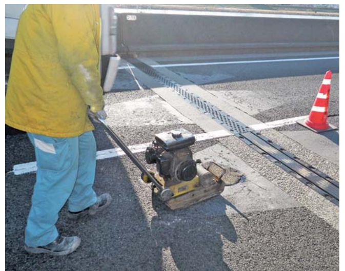
Emergency repair work
