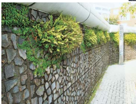
Greening of Yoyogi Parking Area wall
