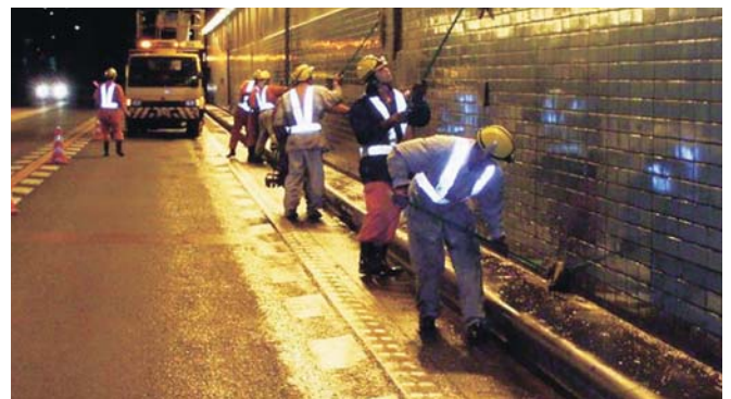
Tile cleaning inside a tunnel
