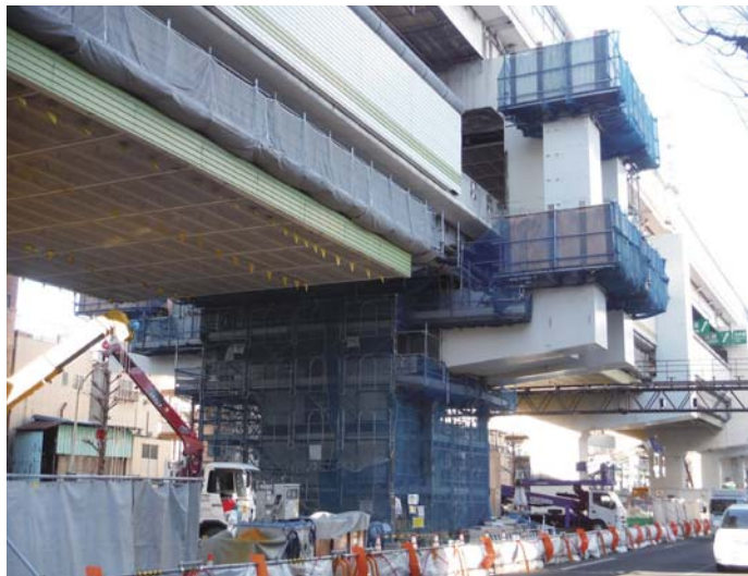
Itabashi Kumanochō Bridge pier work
