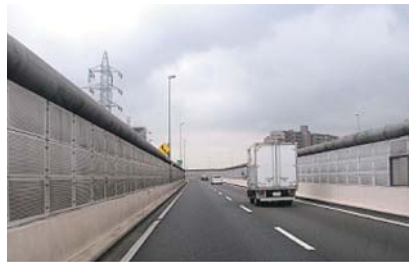
Noise barriers on the expressway
