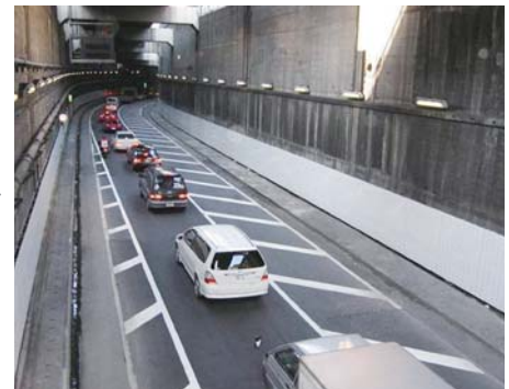
Installation of white tile panels on the wall of Chiyoda Tunnel on the Inner Circular Route
