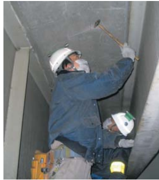
Detailed inspection work
