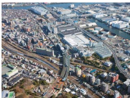
Northern Route Complete view of Namamugi JCT
