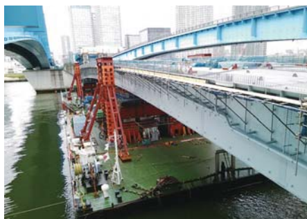
Harumi Route Lift-up barge construction
