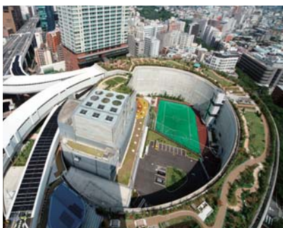
Full view of Ohashi Junction rooftop
