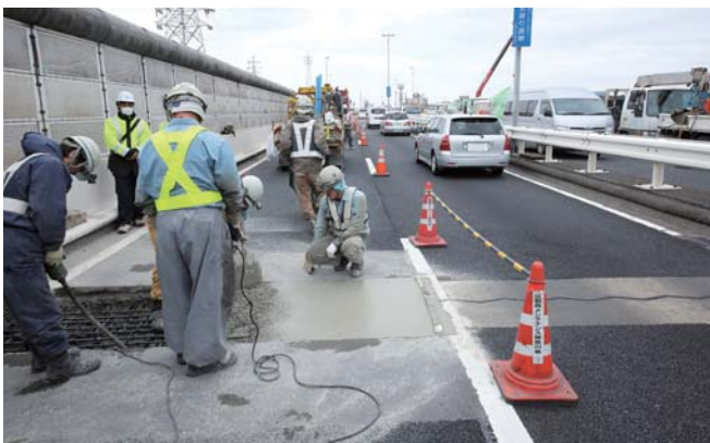
Eliminating expansion joints
