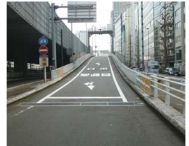
Measures against pedestrian entry (Shibuya Exit of Route 3 Shibuya Line)
