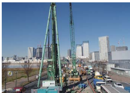
Harumi Route Foundation construction
