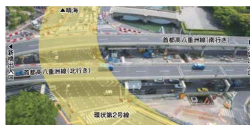
Range of Circular Route 2 renovation
