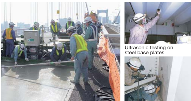
Laying down SFRC pavement as a plate deck fatigue countermeasure
