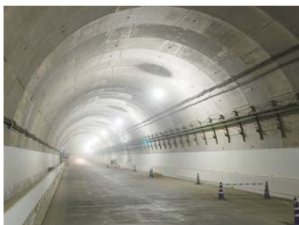
Northern Route Shield tunnel interior
