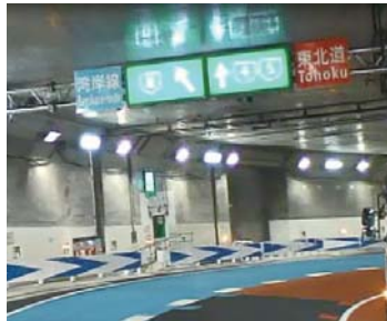
Signboards and road surface classified by color according to direction of travel (Ohashi JCT)
