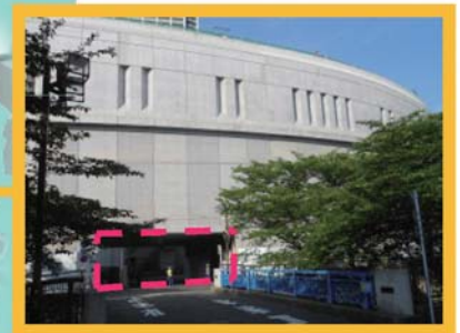
Parking Lot Entrance
