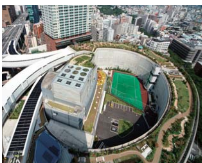
Full view of Ohashi Junction rooftop
