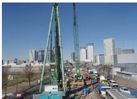
Harumi Route Foundation construction
