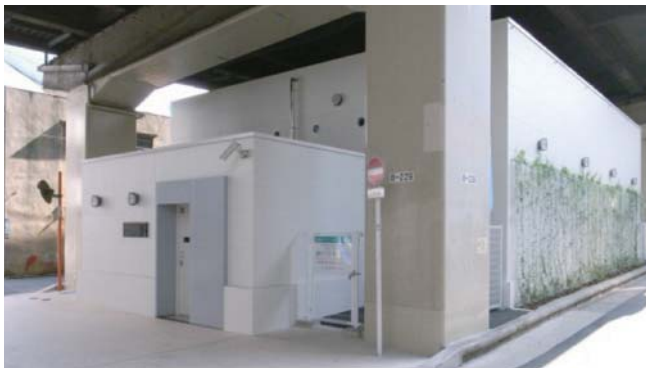
Shutoko Storage Room at Ebisu
