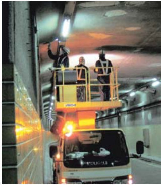
Tunnel inspections using boom lifts
