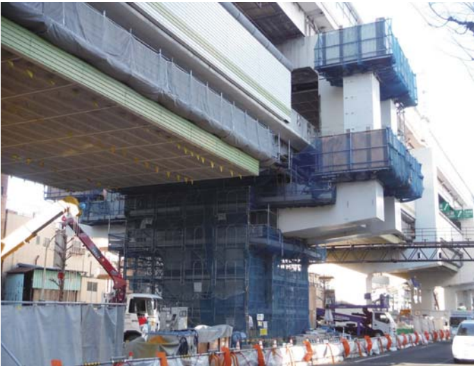
Itabashi Kumanochi Bridge pier work
