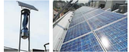
Power generating equipment that uses natural energy (Yoyogi Parking Area)
