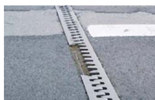
Expansion Joint Replacement
