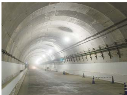
Northern Route Shield tunnel interior
