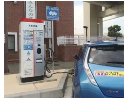
Fast charger for electric cars (Daikoku Parking Area)
