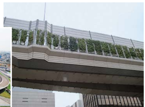
Greening of girders at Nishi-Shinjuku Junction
