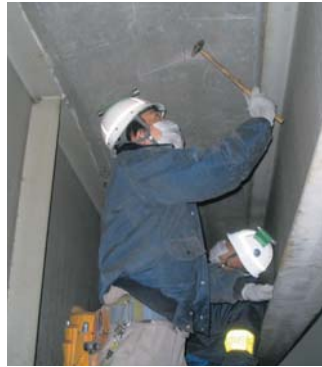
Detailed inspection work
