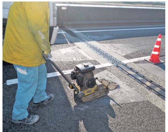
Emergency repair work
