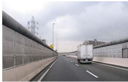
Noise barriers on the expressway
