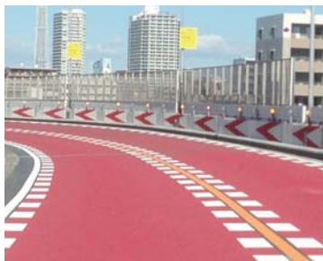
Colored warning pavement (Around Kiba of Route 9 Fukagawa Line)
