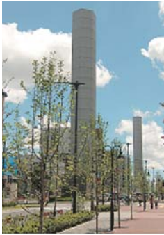
Yamate Tunnel ventilating tower.
