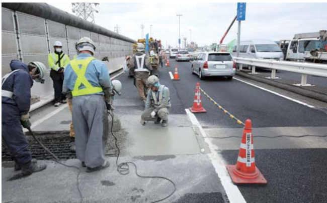
Eliminating expansion joints
