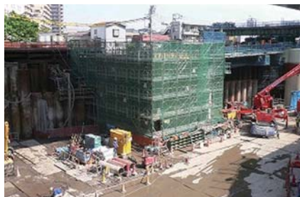
State of work on the ramp at Oji-minami
