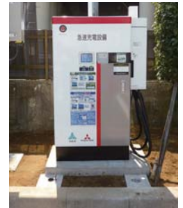
Electric Car Fast Charger (Kawaguchi Parking Area)
