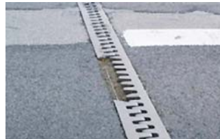
Expansion Joint Replacement
