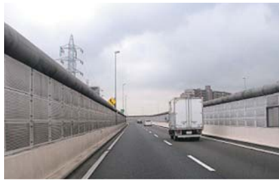
Sound barrier above the wall of the expressway.
