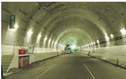
State of construction on the main route shield
