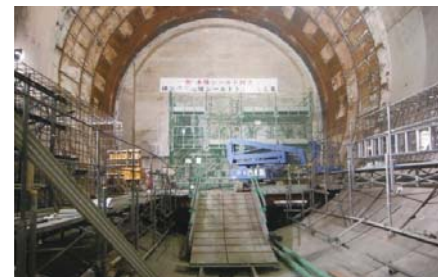
State of completion of shield
