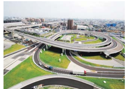
Greening of Daishi Junction.
