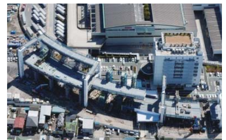
State of construction at Namamugi junction
