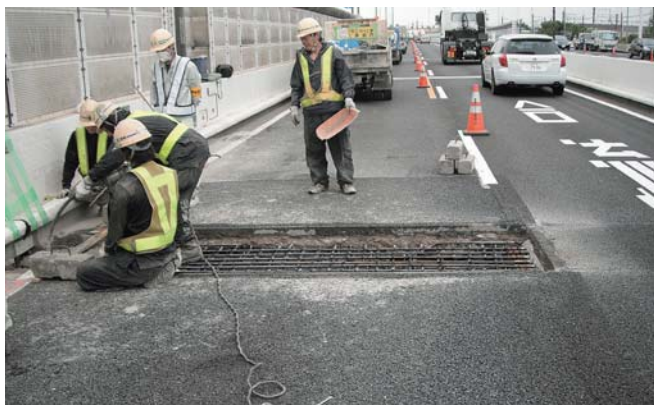
Eliminating expansion joints along the Yokohane Line
