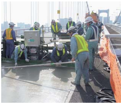
Laying down SFRC pavement as a plate deck fatigue countermeasure
