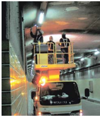
Tunnel inspections using boom lifts
