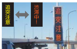
Tailback Rear-end Collision Countermeasure (LED panel)
