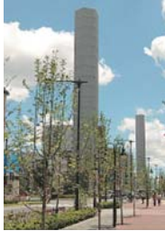
Yamate Tunnel ventilating tower.
