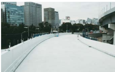
State of construction at Oi junction
