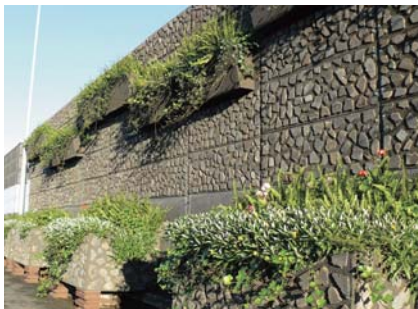
Greening of viaduct wall near Urayasu on the Bayshore Route.
