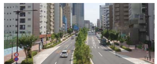
After work on No. 6 Circular Route
