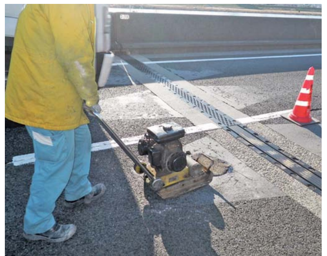
Emergency repair work
