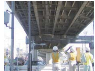
Inspecting under Viaducts
