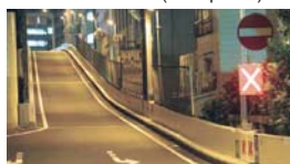
Measures to prevent Mistaken Pedestrian Entry (LED “no entry” panel)
