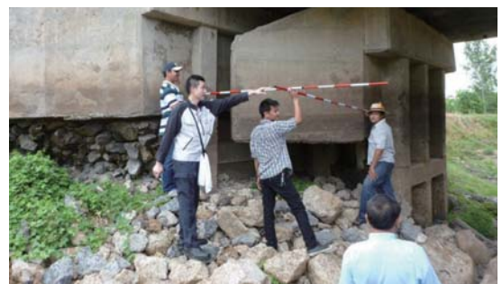
On the job bridge inspection training for overseas technicians (Thailand) as part of our overseas consulting business activities
