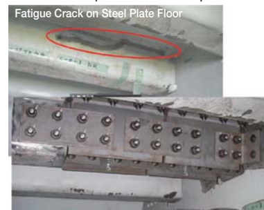
Crack Repairs using Reinforcing Plating
