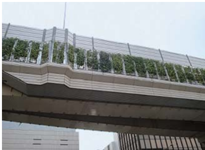
Greening of girders at Nishi-Shinjuku Junction.
