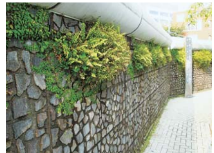
Greening of Yoyogi Parking Area wall.
