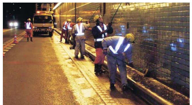
Tile cleaning inside a tunnel
