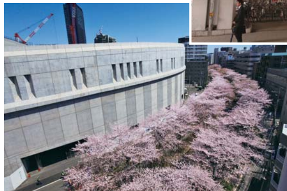
Ohashi Junction wall surface
