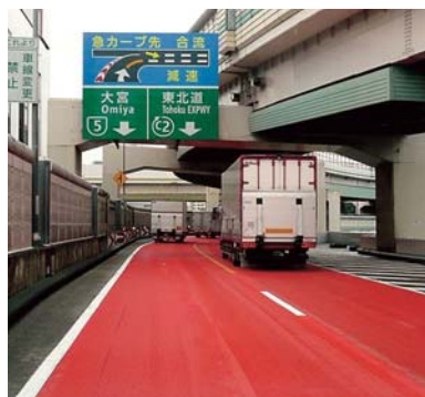
Road Curve Safety Measures (Attention-grabbing colored road surface and large warning signs)
